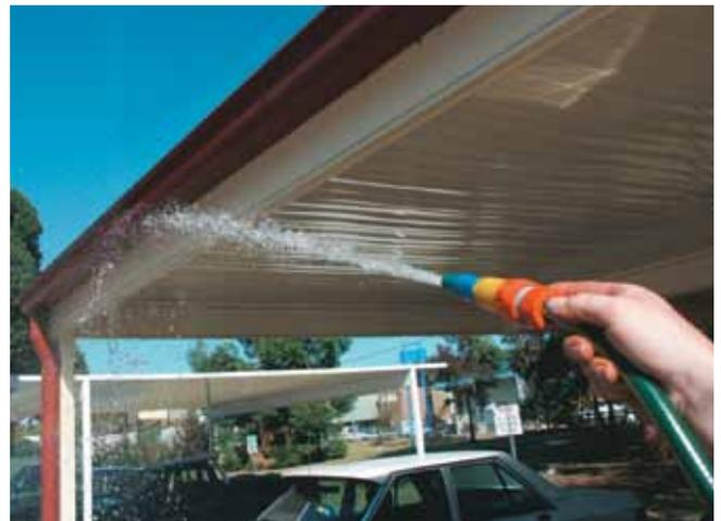
**Use a hose to rinse the underside of gutters & roofs**
