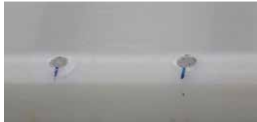
Figure 6: Pre-drill holes of upper translucent sheet at TRIM-KLIP bracket.
