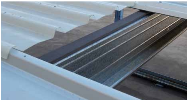
Figure 5: Upper translucent sheet with packer at support.
