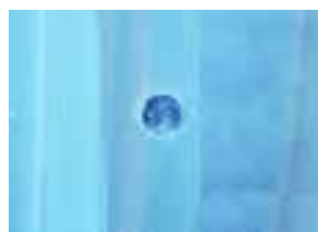
Figure 3: Pre-drill hole at lower translucent sheet at TRIM-KLIP joint.
