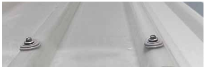
Figure 2: TRIMDEK and Ampelite 5-Rib lapping
