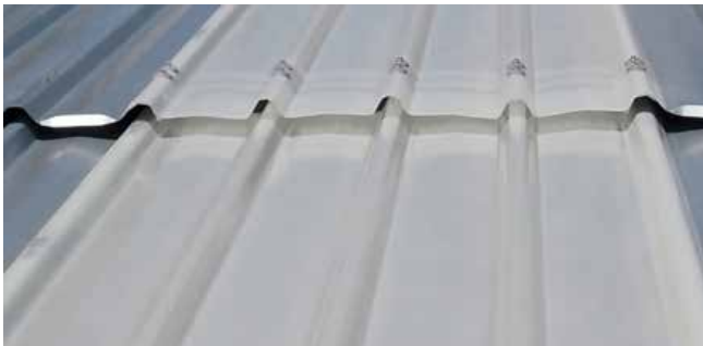
Figure 1: Finished installation of Ampelite at TRIM-KLIP joint
