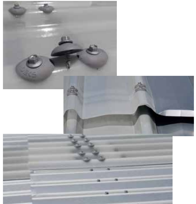
Figure 7: Upper translucent sheet fixed to TRIM-KLIP brackets
