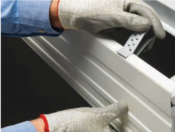
Step 1: Preparing to attach spring clip
