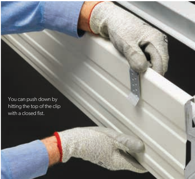
Step 2: Final position of spring clip
