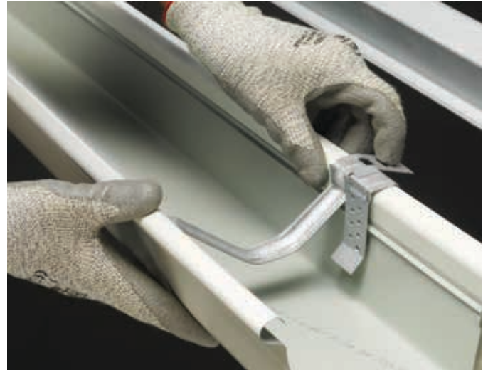
Step 3: Attaching the gutter overstrap
